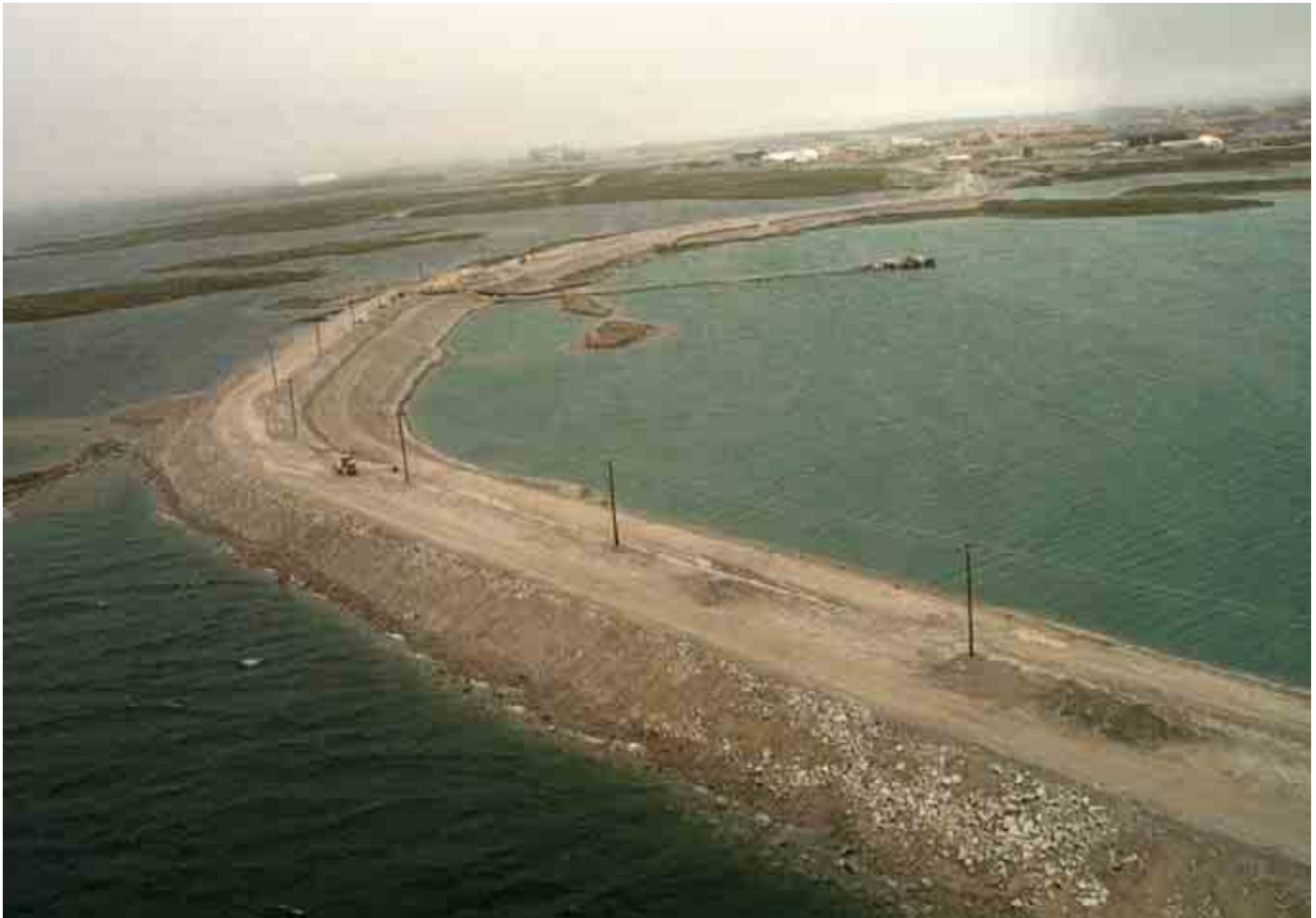
Dike completed in summer 2002
