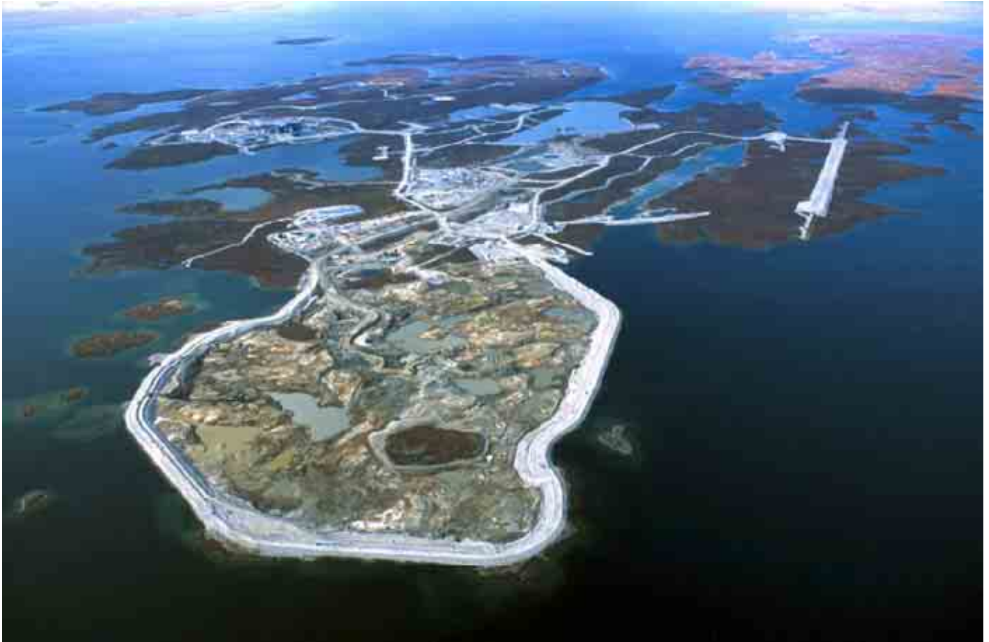
Diavik end of Sep 2002: dewatering finished
