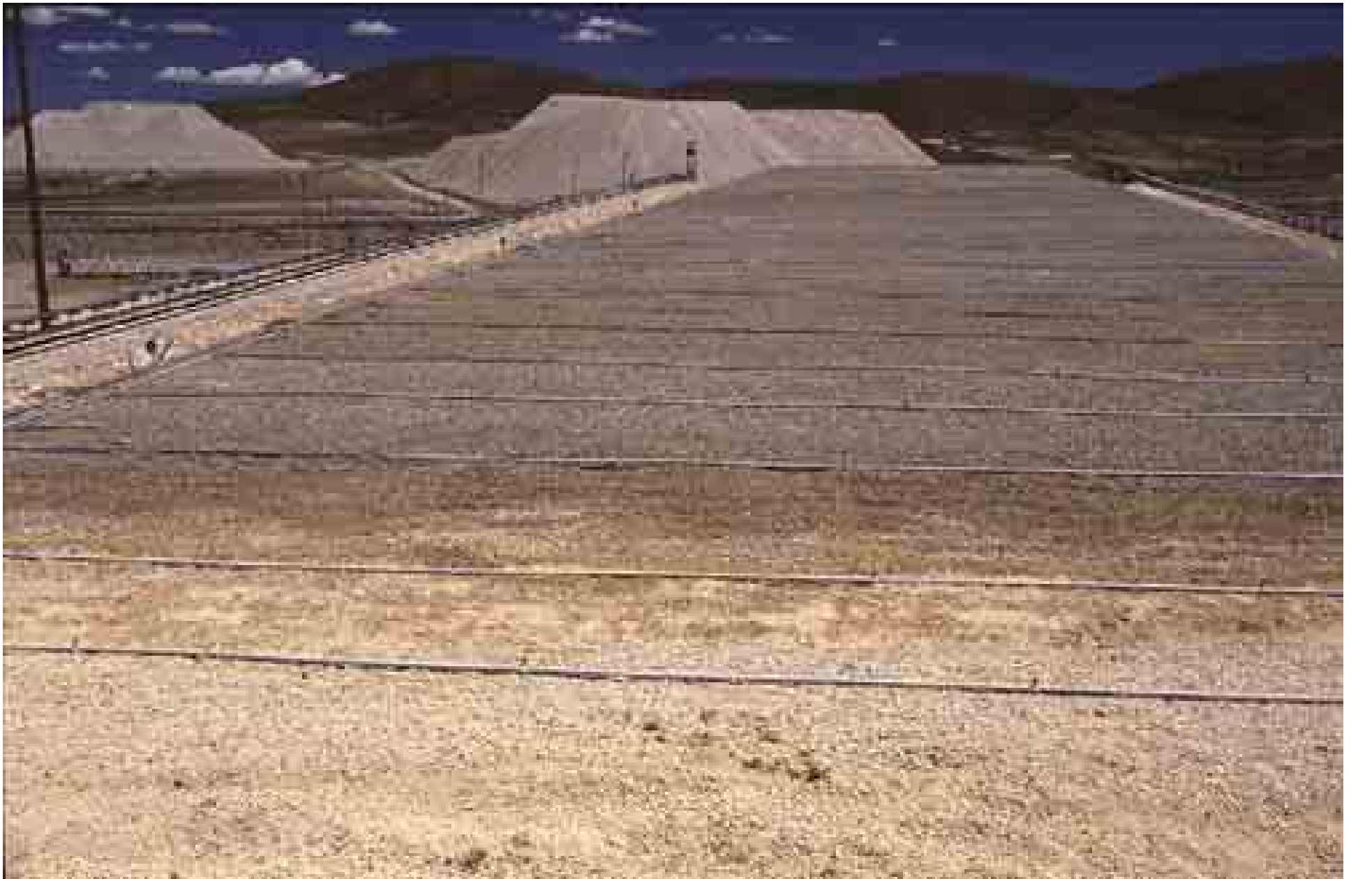
Kori Kollo, Bolivia: Leach pads
