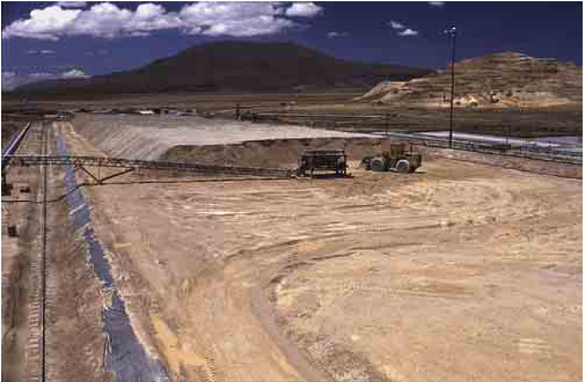
Kori Kollo, Bolivia: Leach pads
