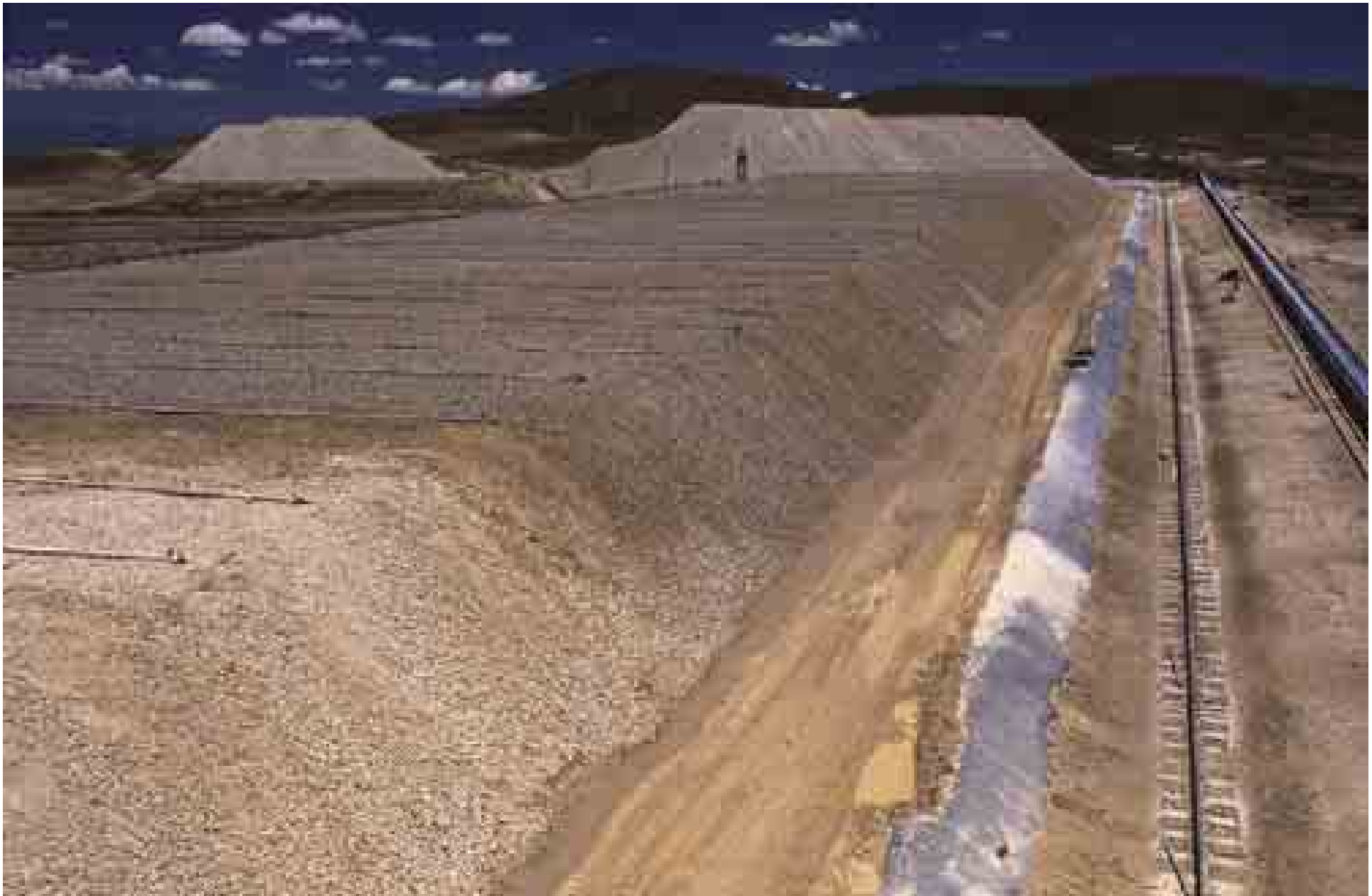
Kori Kollo, Bolivia: Leach pads
